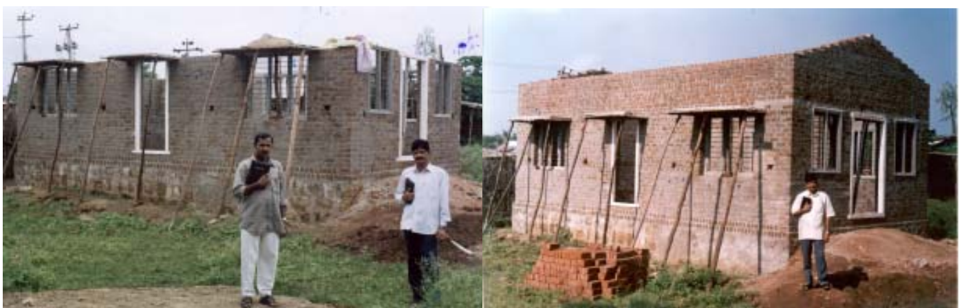
Church under construction at Prashanthnagar
