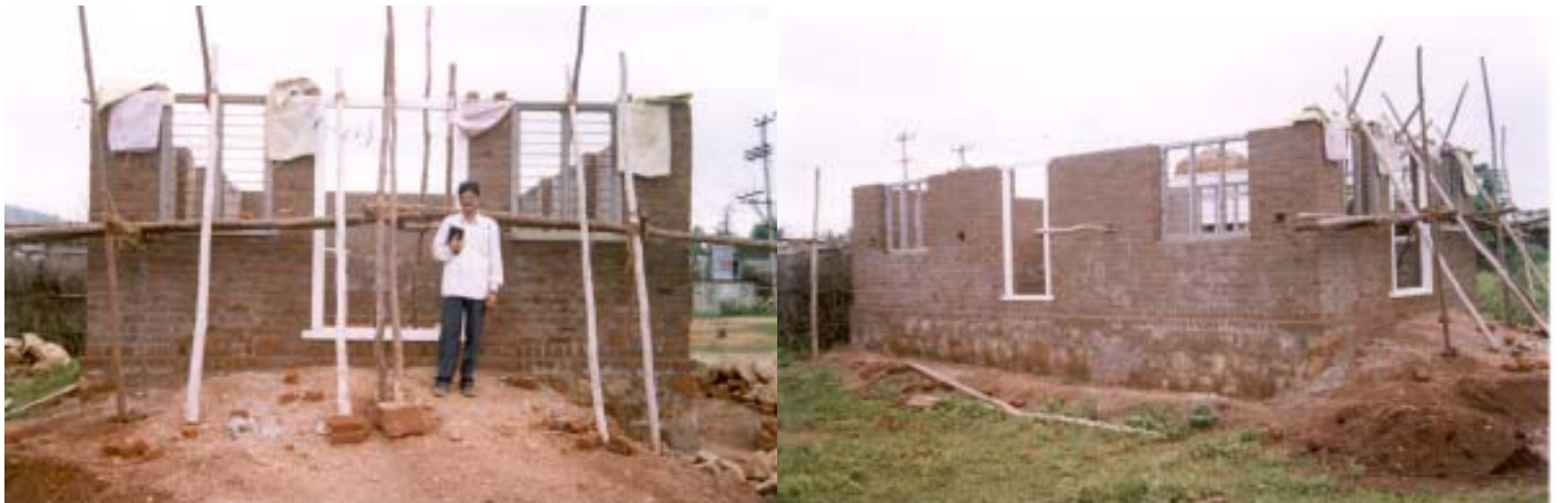
Church under construction at Paloncha
